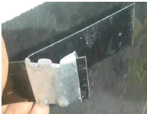
06. Figure 15: Location of the strap failure in the place of the notches in beam 06.
