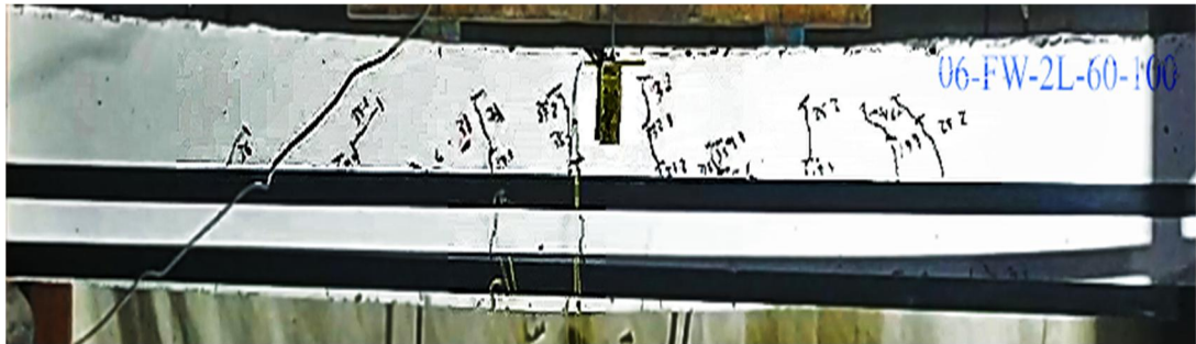
Figure 14: Crack pattern of beam 06.
