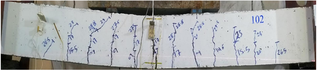
Figure 9: Crack pattern of the beam 102.
